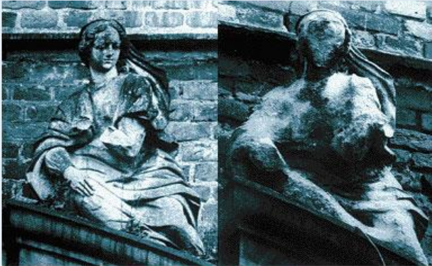
How acid rain affects stonework. The picture on the left was taken in 1908. The picture on the right was taken in 1968
